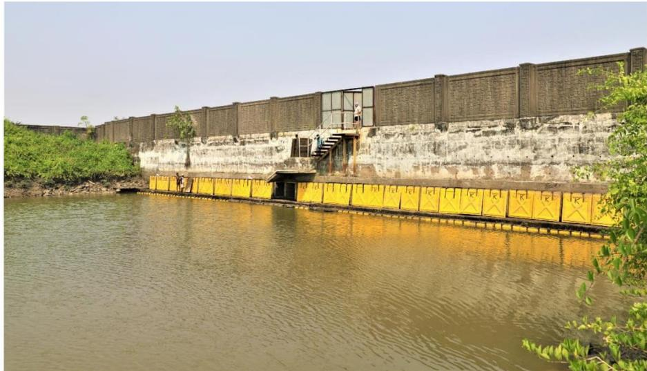
**Image 1:** Tide gate on the creek at Panje Wetland. Image shows upper 35 flip valves while lower 35 valves are submerged. Currently these flaps are open allowing tidal water to flood the wetland. The closer of these flaps will kill the entire wetland
