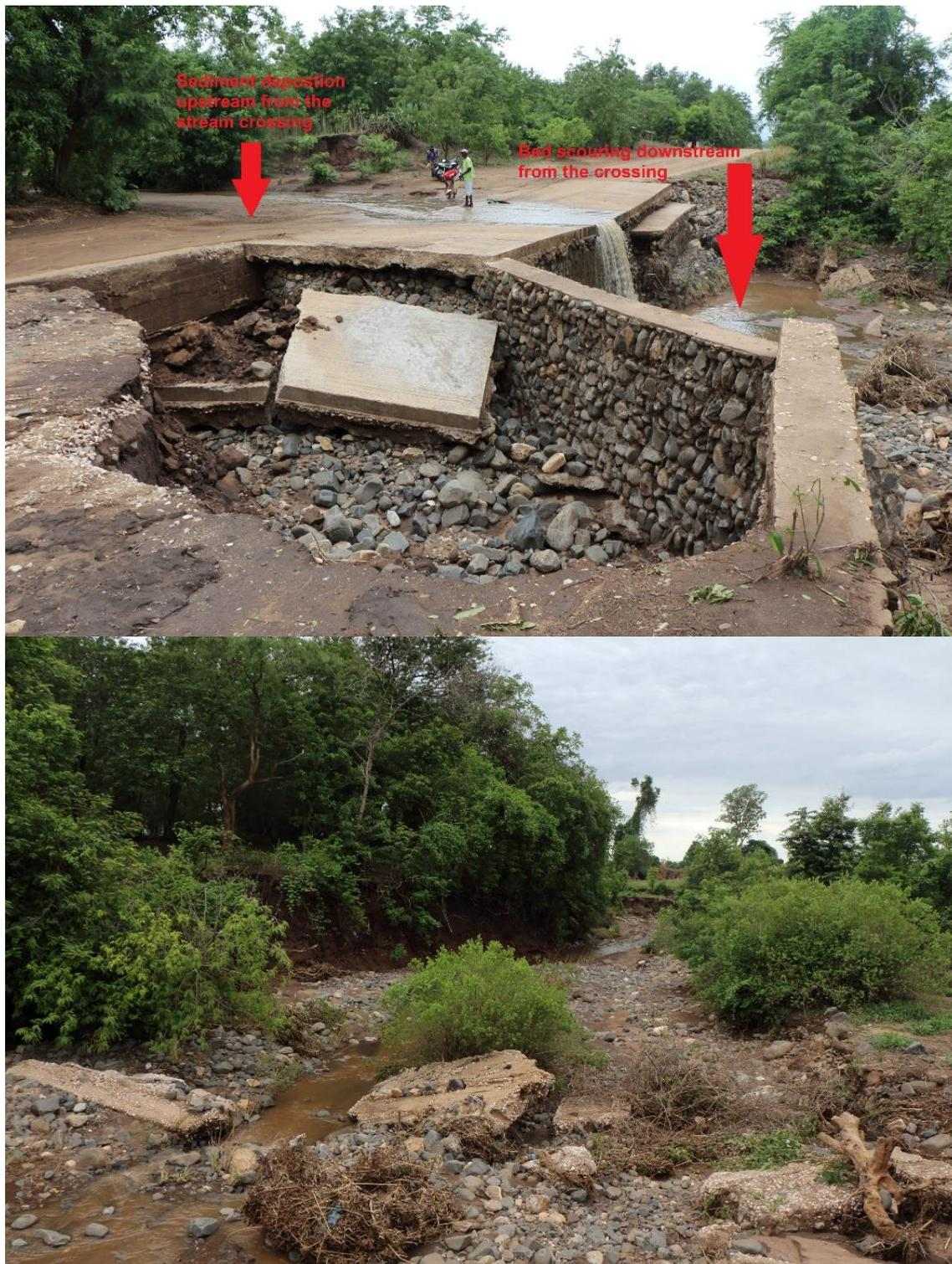
Figure 17. High run-off and eroded soils end up in the rivers, clogging and accumulating at obstructions, and resulting in severe damage to infrastructure, the river bed and inevitably biota (S16.16474 & E34.98224, 18 January 2016, G Diedericks).
