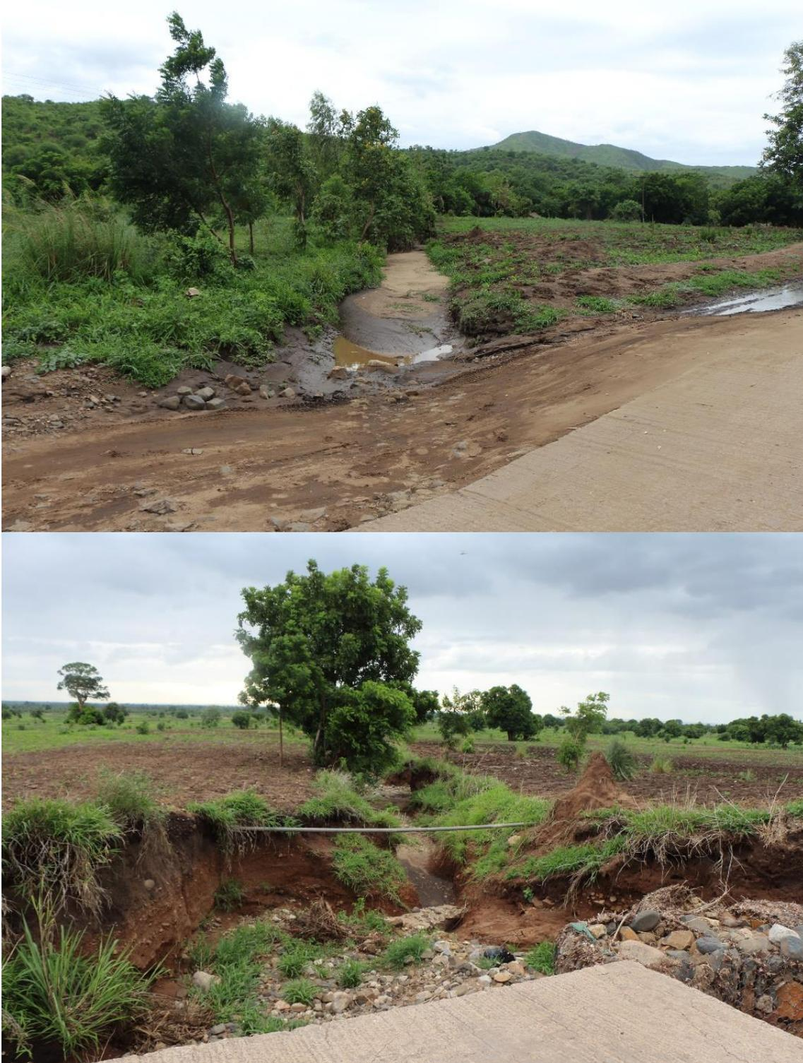
Figure 18. Agricultural activities in the riparian zone, with no riparian buffer zone is evident up- and downstream from the crossing. Eroded soil deposited into the stream deposits upstream from the crossing, and the “higher” water level during flood events increases erosive capacity, which is evident from the bank and bed scouring downstream from the crossing (S16°5'47.5" & E34°54'43.52", 18 January 2016, G Diedericks).
